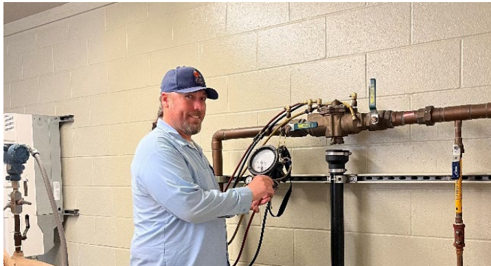
CHWD Staff Performing Testing A Backflow
