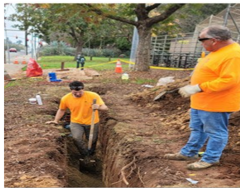
CHWD Staff Installing A Service line
