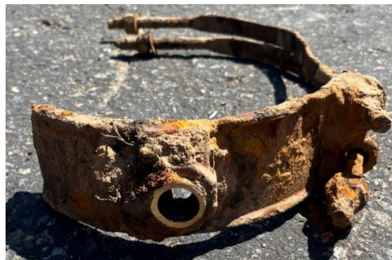
Cast Iron Saddle Removed from Field
