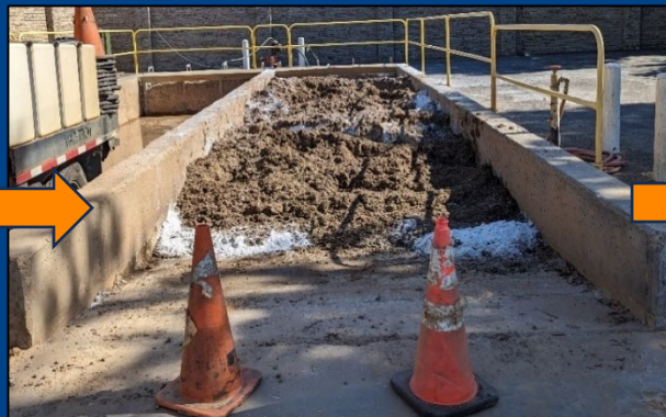
The perlite is mixed into the spoils using an auger attachment on a backhoe. The result is a drier, stackable dirt.
