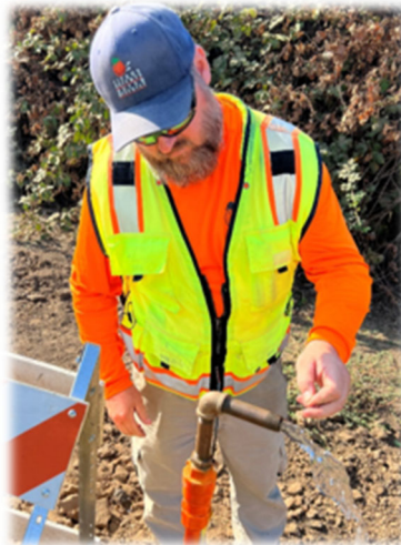
CHWD Staff Completing Testing for Chlorine Residual on a Newly Installed Water Main
