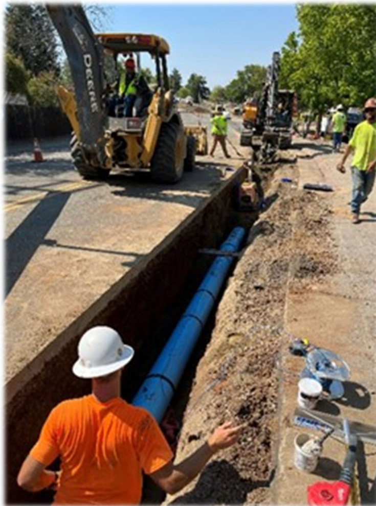
Installation of Water Infrastructure
