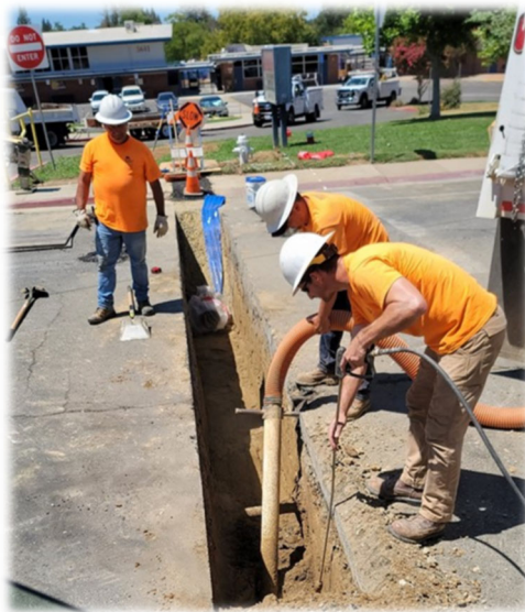
CHWD Staff Performing Work for Skycrest School Water Main Project
