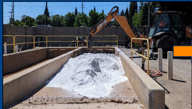
Perlite added to the vacuum basin.
