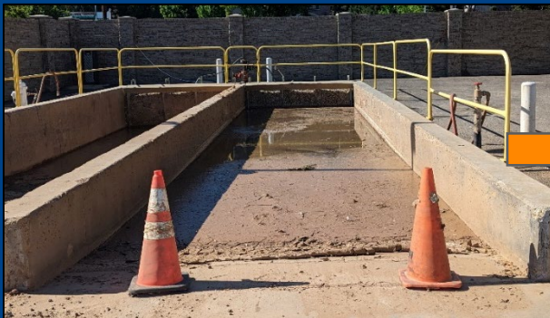
Vacuum excavation slurry is discharged into the vacuum basin.
