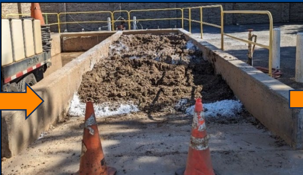
The perlite mixed into the slurry. The result is a drier, stackable dirt.
