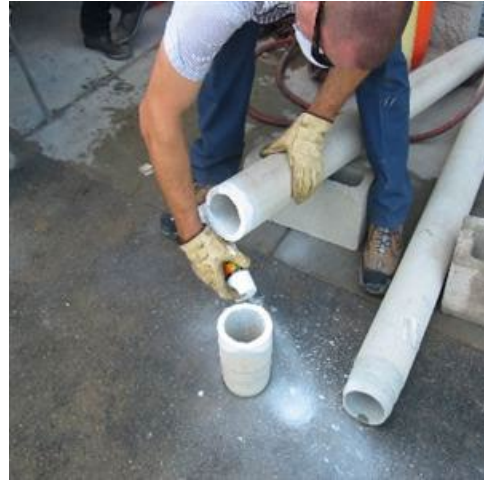
Worker painting the end of asbestos pipe to prevent fibers from becoming airborne (stock photo)
