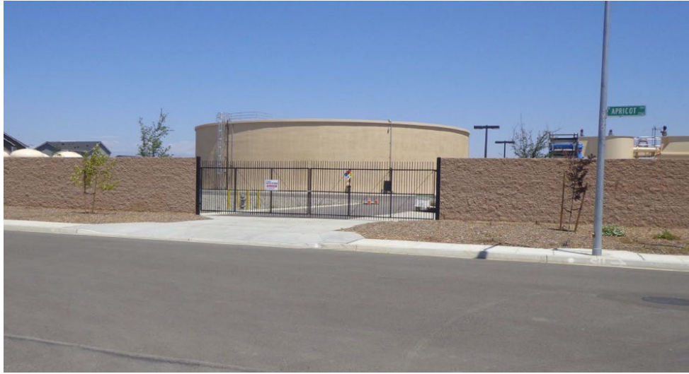
Figure 8: Pre-Stressed Concrete 5-MG Tank, Basic Paint, Fresno County
