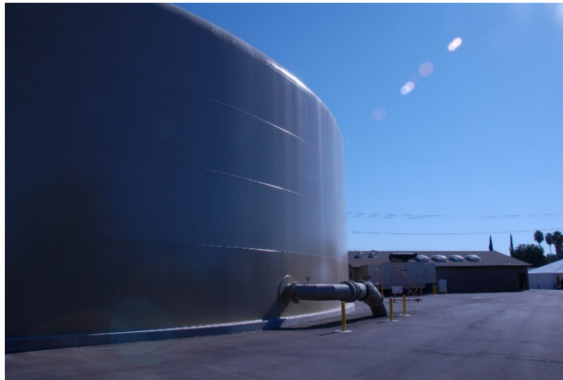
Figure 7: Welded Steel 5-MG Tank in Sacramento
