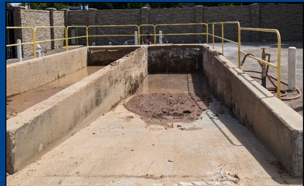
The storage basin can then be cleaned out with the front bucket of a backhoe and the dirt can be disposed of.
