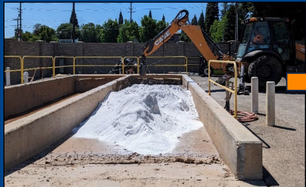
Perlite is added to the storage basin.
