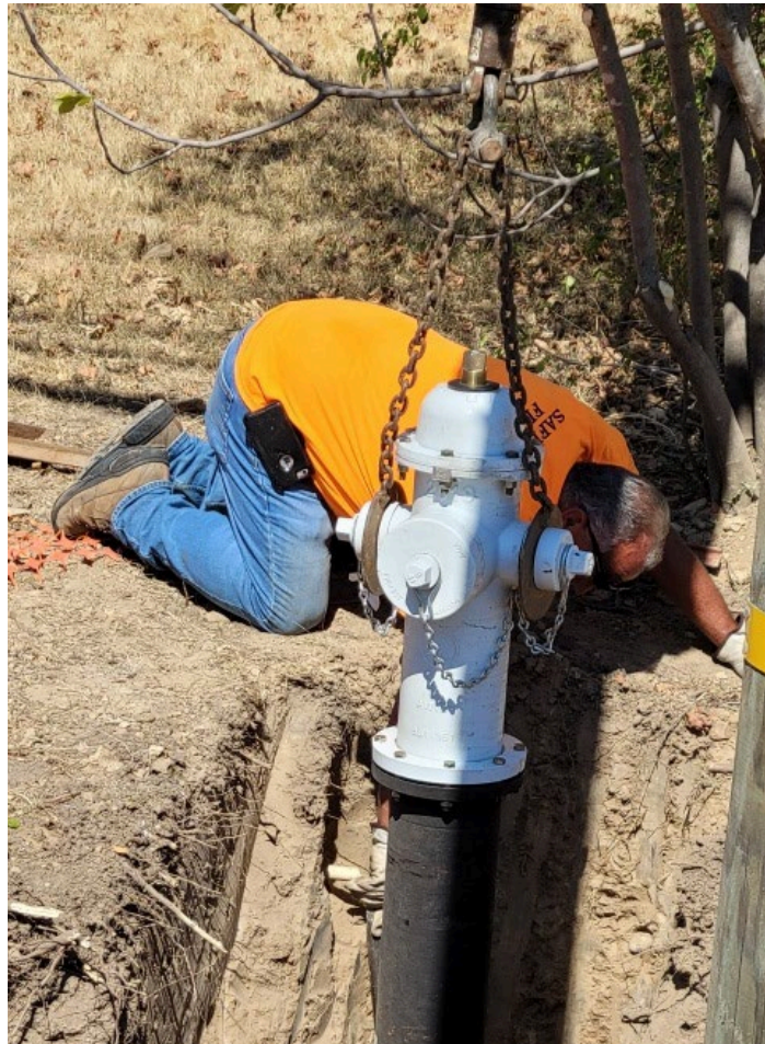
Photo: CHWD fire hydrant installation
