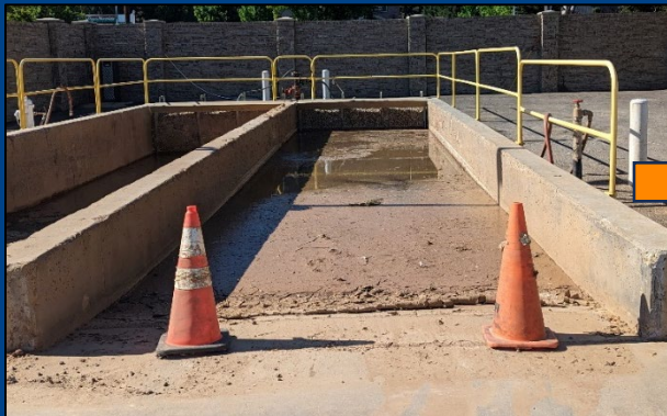
Vacuum excavator spoils are dumped into the storage basin.
