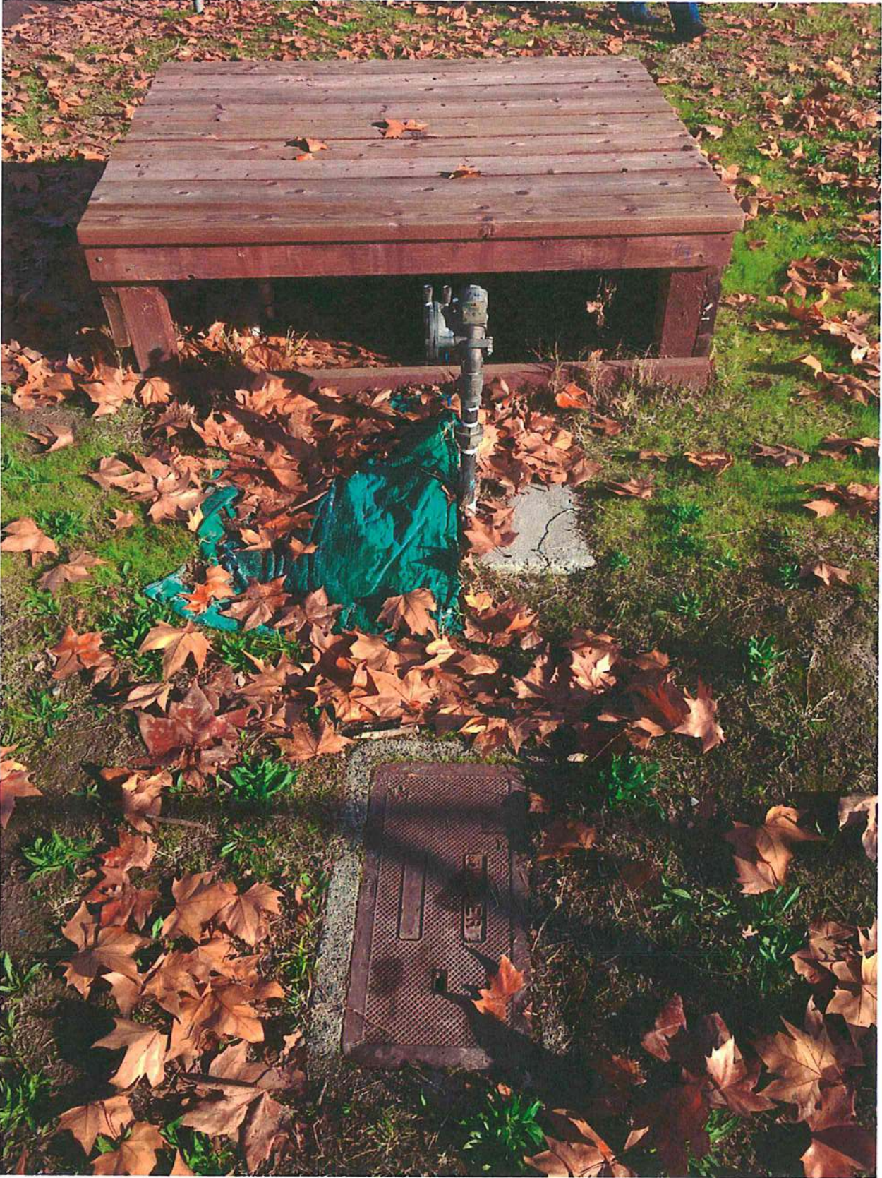
Item #11 – Water Meter and Backflow
