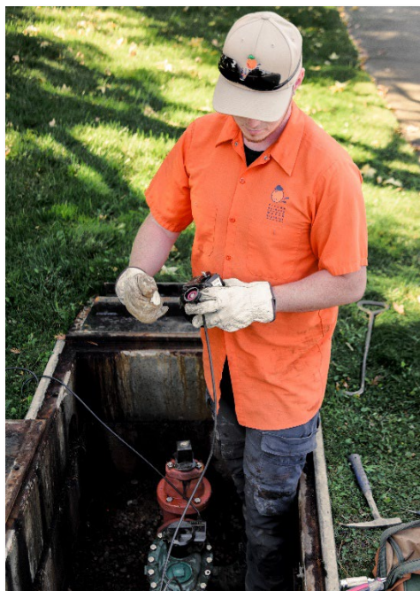
CHWD Staff Servicing a Water Meter
