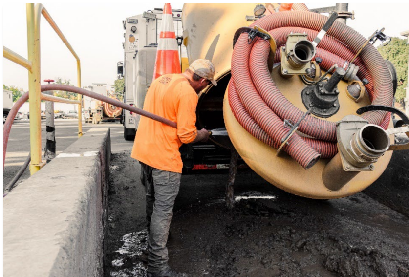
CHWD Staff Washing Material Out of Vacuum Excavator Holding Tank
