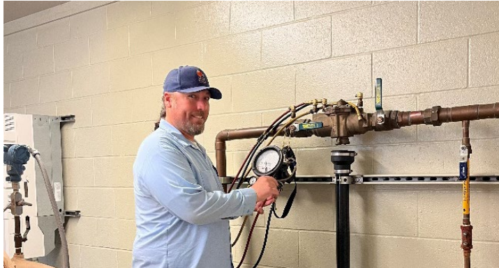
CHWD Staff Performing Testing A Backflow
