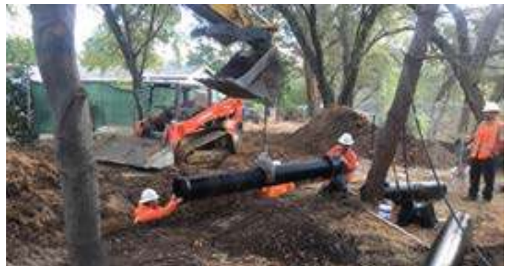
Workers shown here are assisting with the installation of pipeline for the Mesa Verde High School Transmission Main Project.
