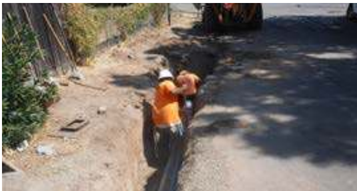
Work progresses on the Baird Way Water Main Replacement Project.
