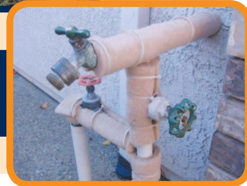
If a pipe becomes frozen, you can thaw it by heating water on the stove, soaking towels in the warm water and wrapping them around the pipes. Use caution when handling hot towels to prevent scalding. Begin thawing nearest to the faucet and turn the faucet on to allow melted water to drip out.
