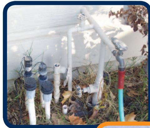
An uninsulated pipe is at risk of freezing and bursting during winter weather. It's also wise to unhook your hose during freezing weather.
