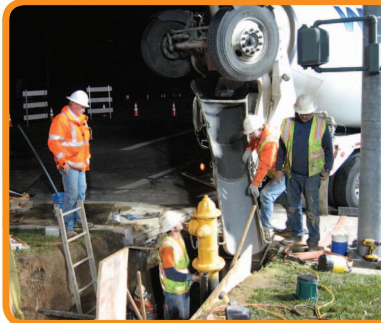
Construction crew pouring concrete as work on the water main replacement wraps up.
