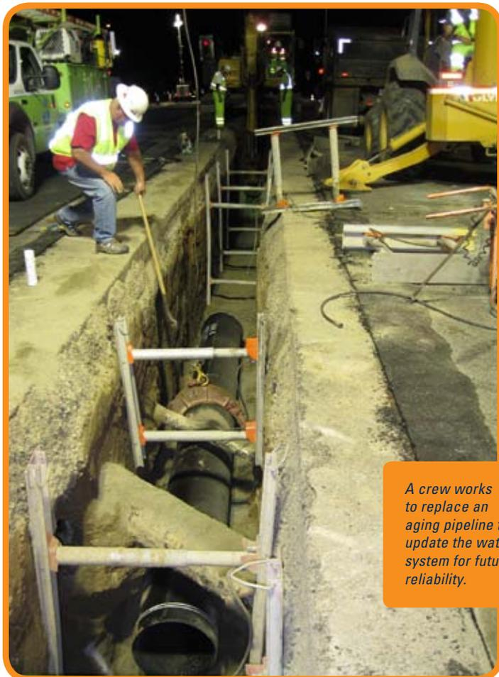
*A crew works to replace an aging pipeline to update the water system for future reliability.*
